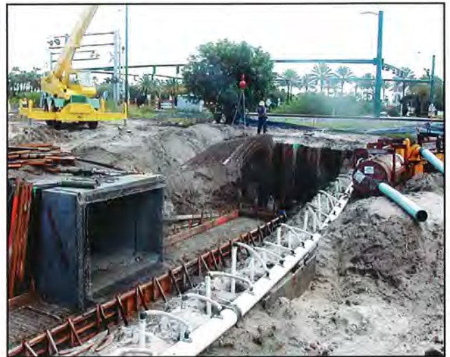
WGI DESIGNED THE EPB-3 CANAL/HOOD ROAD BOX CULVERT
