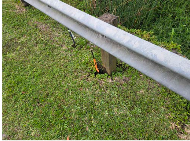
Ground subsidence adjacent to roadway safety barrier — evidence of underlying CMP collapse.
